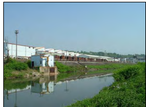
AK Steel Corporation Butler Works
