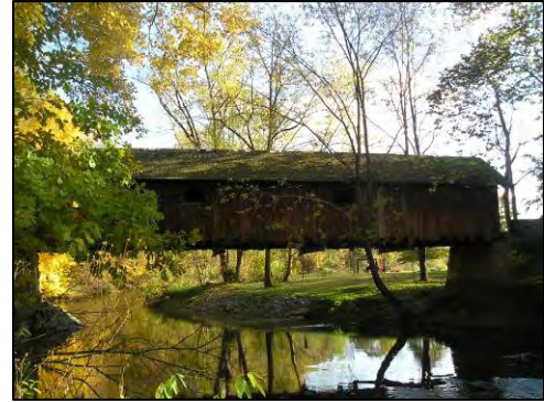
Woolslayer Bridge extends 75 feet across Brush Creek in New Sewickley Township, Beaver County
